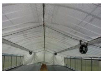
Solar Screen/ Ventilation fans
